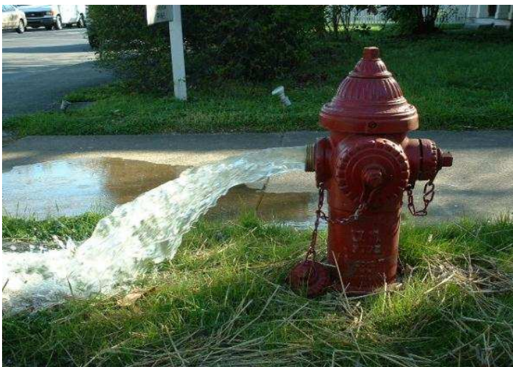
Top: Picture of a flushing hydrant.
